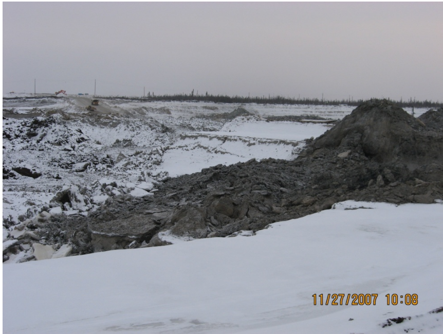
On site picture of the failed slope
