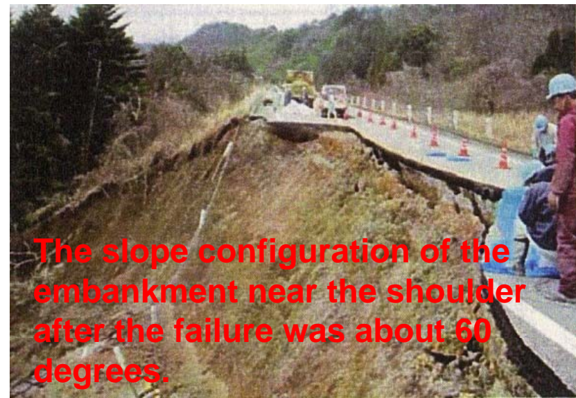
Embankment failure at site T6
