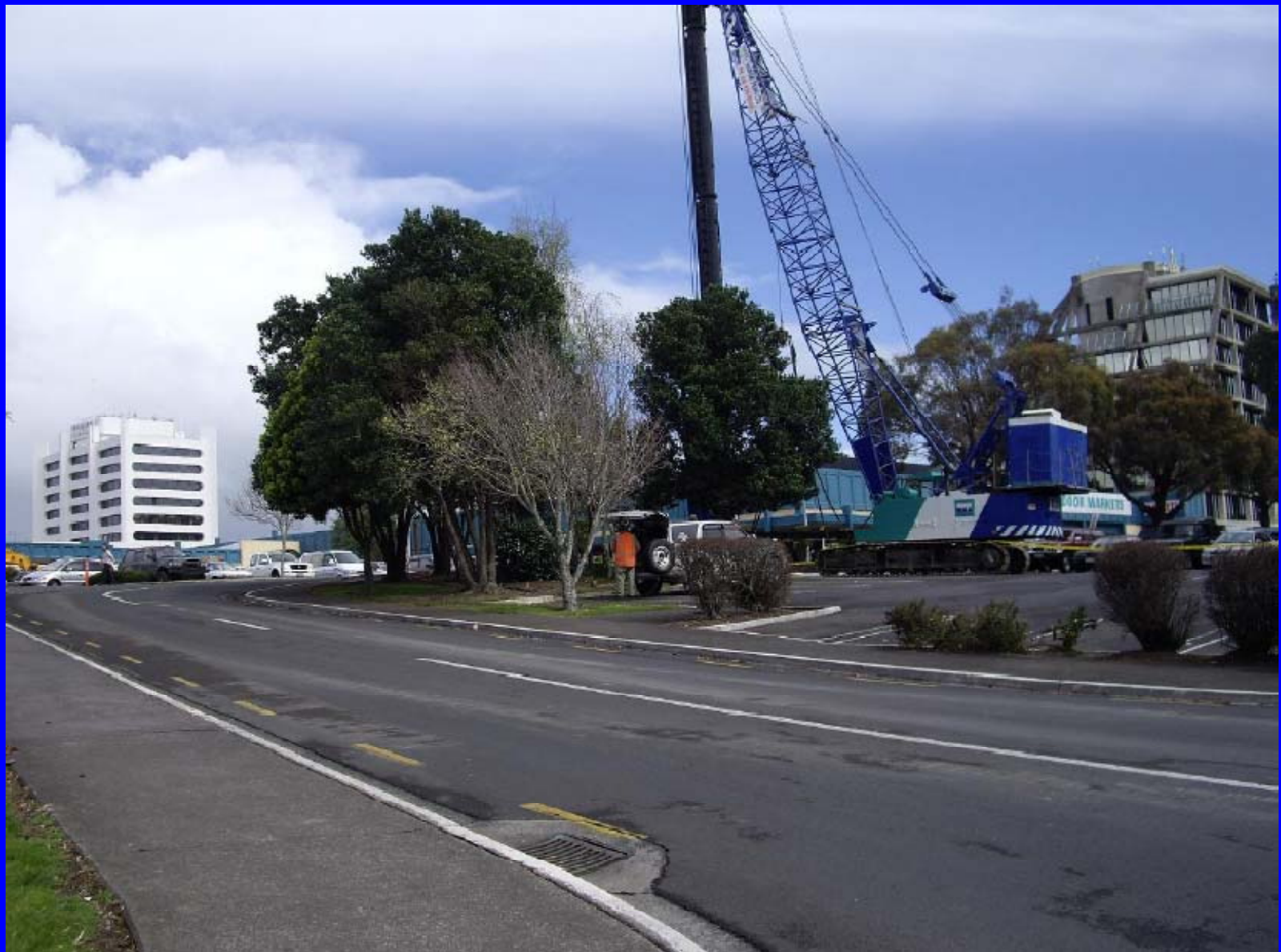
PDA testing at Test Pile 3
